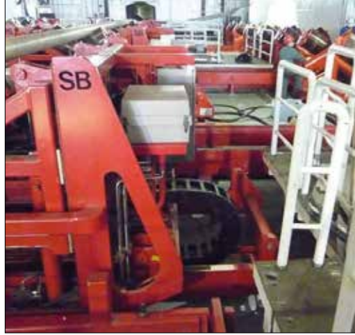
... on pipe handling equipment.
